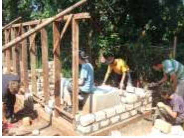
Constructing toilet block
