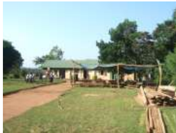
Classrooms at Bukeka Centre
