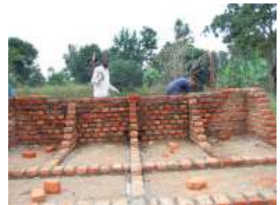
Moses (local craftsman) & Calum working on wash-house
