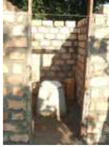
Addition of toilet
